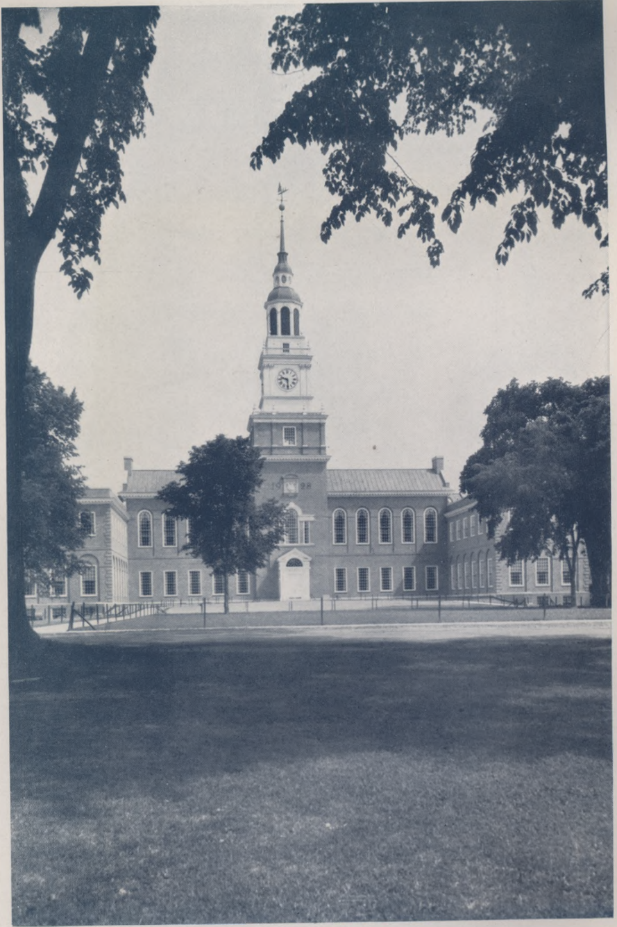
BAKER MEMORIAL LIBRARY DARTMOUTH COLLEGE, HANOVER, N. H. CONTAINING OUR HEAVY CHIME OF SIXTEEN BELLS
