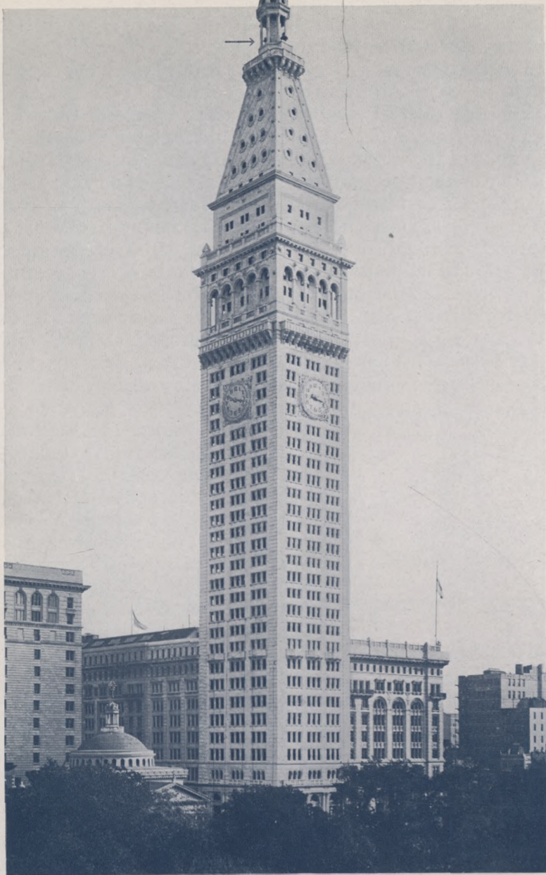
METROPOLITAN LIFE INSURANCE BUILDING. TOWER 700 FEET HIGH. ARROW SHOWS WHERE BELLS ARE PLACED.
