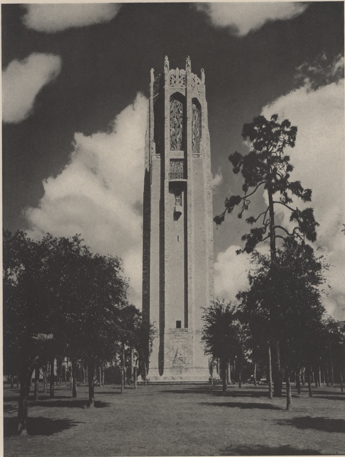
The south front of the Singing Tower, with sun-dial at base. The ashlar is Coquina rock, a salmon-pink coral formation. Georgia Marble is used for the base, buttresses and top, with gray Creole at base and shell-pink Etowah above.
