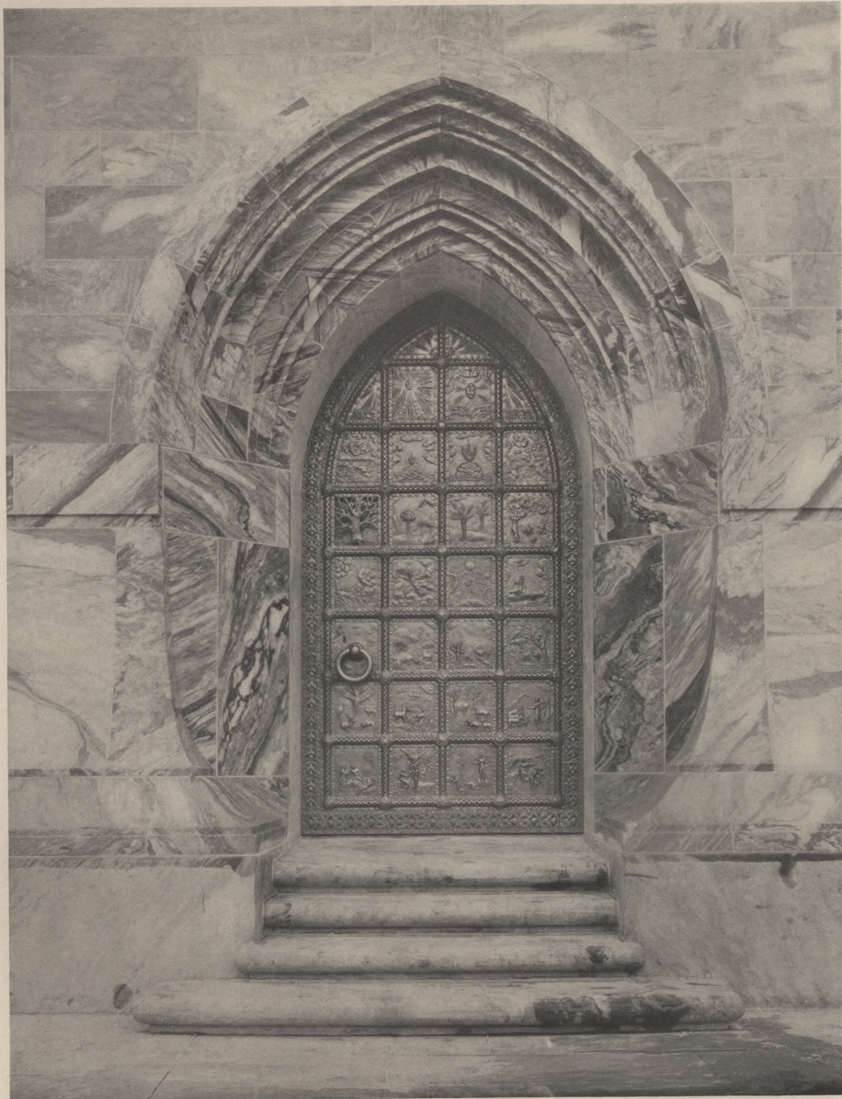
The great Golden Door which is the sole entrance to the Tower. The door was designed and hammered out in repousse brass by Samuel Yellin, and represents the story of the Creation.
