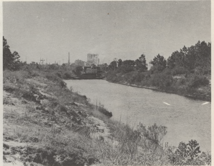
Enormous amounts of wood and wood-chips, left, are required for the huge St. Joe Paper Company mill, which operates around the clock. Right, an eighteen and one-half mile canal was dug between the Chipola River and Port St. Joe in the 1950's, supplying fresh water for the paper mill and for the town.
