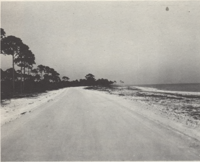
Alfred I. duPont spurred the building of roads in northwest Florida. This is the Gulf Coastal Highway, U.S. 98, skirting St. Joseph Bay near Port St. Joe.
