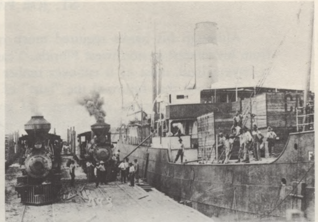
In 1920 Port St. Joe was a busy sawmill town, from which shiploads of lumber went to Eastern ports and to Europe. When Edward Ball purchased 240,000 acres of cut-over land in the surrounding area in 1933 for Alfred I. duPont the sawmill was closed down and the town was dead.
