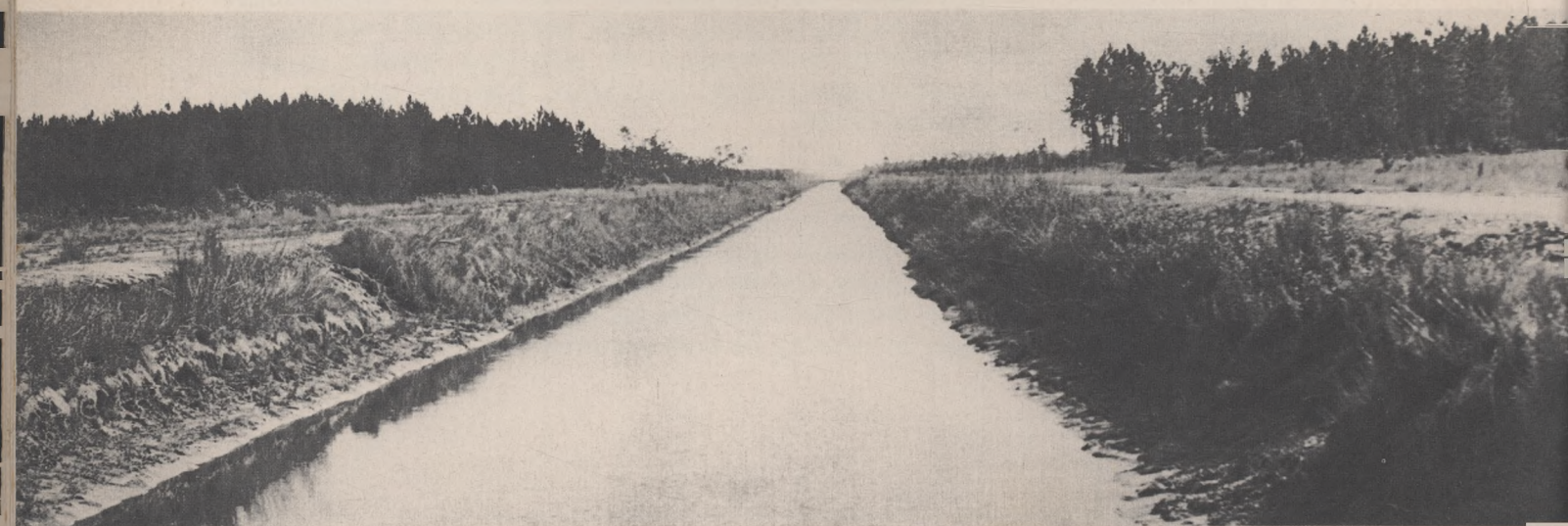
An 18½-mile company-built canal solved the problem of fresh water for the mill
