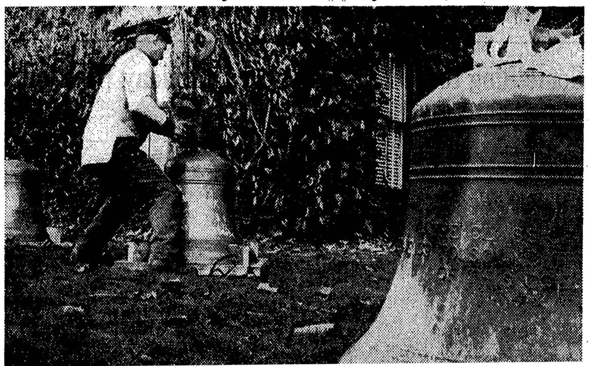
A workman adjusts a crane hook on one of the new bells that will be hoisted to the tower atop Wesleyan University's South College. Bell in foreground is one of the original eleven bells that were built in 1916 and installed two years later in the tower.
